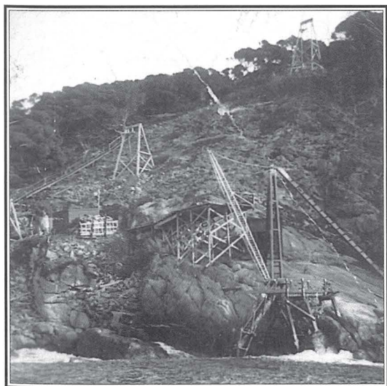
Steel Derrick, landing ladder, flying fox and trestles from timber platform to summit on a calm day. (Photograph Syd O'Neill)
